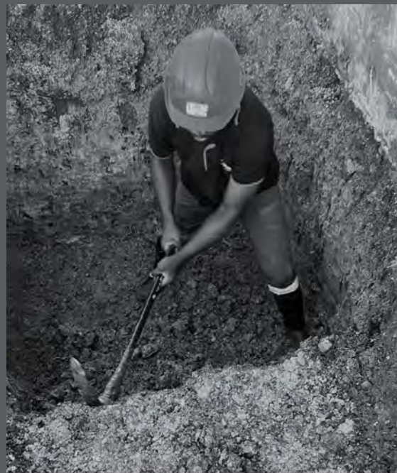
Figure 2. Construction underway in Palm Ridge.
